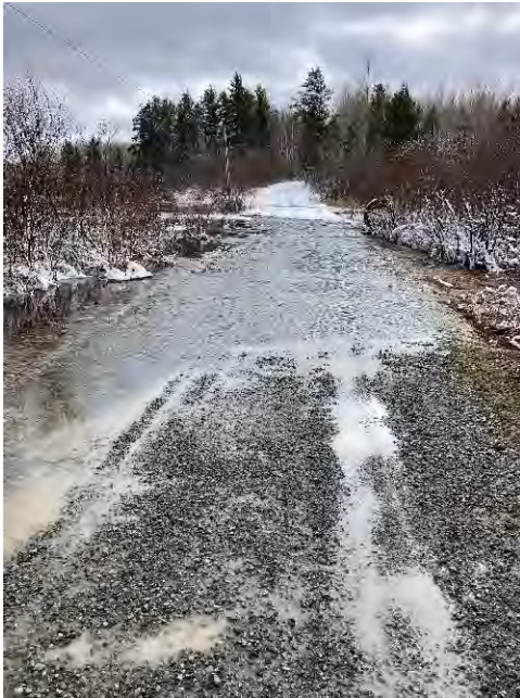
Photograph 8: Road being overtopped during flooding resulting in damage to the road.
