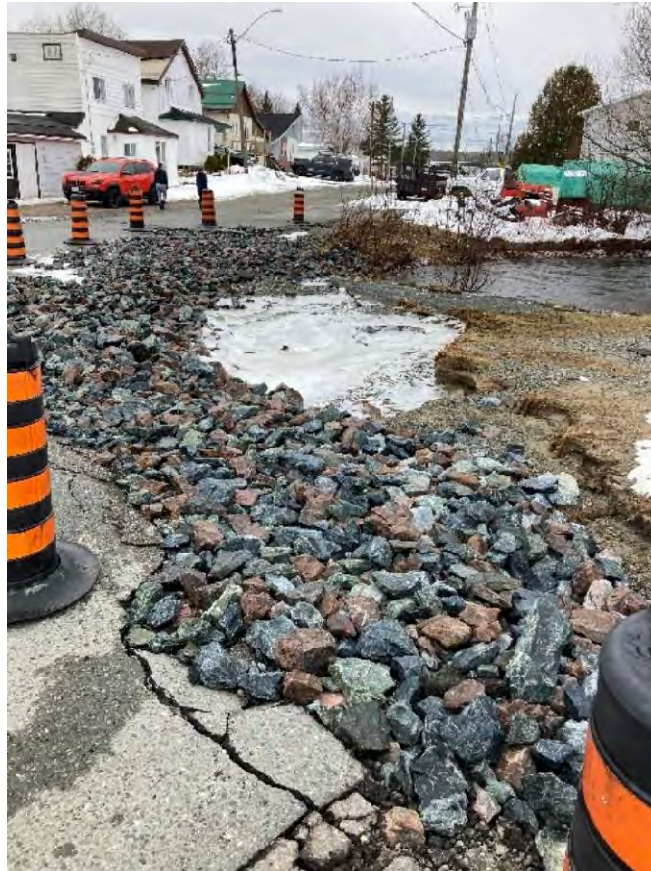
Photograph 6: Rip-Rap placement after road was eroded during flooding
