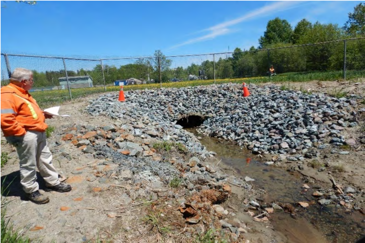
Photograph 1: Rip rap Placement. Looking north east.
