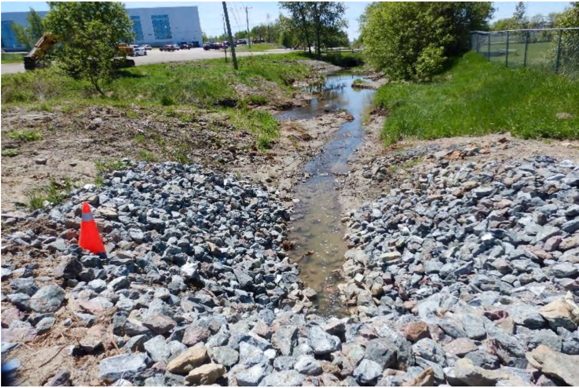
Photograph 2: Ditch shown was cleaned out with excavator after flooding .Looking south west.
