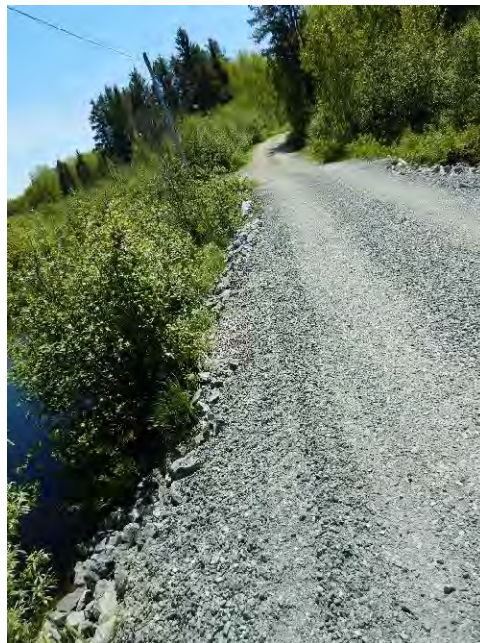
Photograph 10: Rip-rap and granular 'A' installed post flooding
